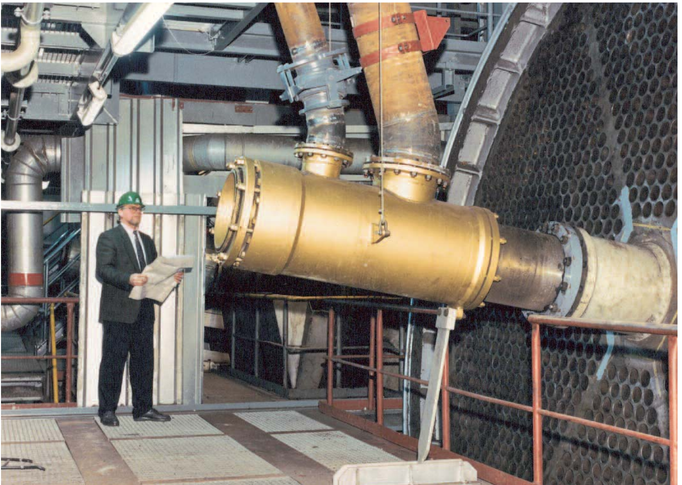
Series H + DC: Especially suited for large steam capacities; available diameters up to DN 350.
